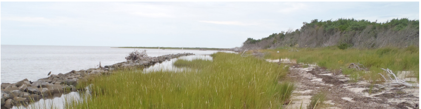
Hatteras, NC. The Durant's Point living shoreline project protects the shoreline from storm surge while providing habitat for many species. Since its construction, the project has weathered hurricanes, a summer of drought, and tropical storms. Photo: N.C. Coastal Federation
