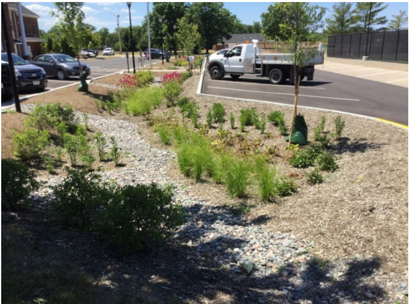
Rain Garden — City Hall in Bay Village, OH
