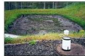
Surface Sand Filter
