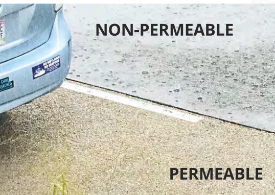
Notice how rainfall soaks into permeable pavement
