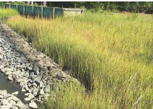
Pine Knoll Shores residential shoreline after restoration
