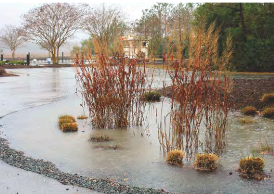
Rain Garden during 1.5" rain
