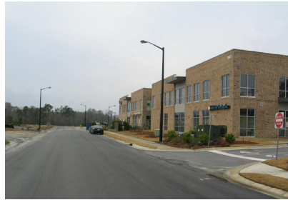
Frontage road with new development along US 17 at Wal-Mart site
