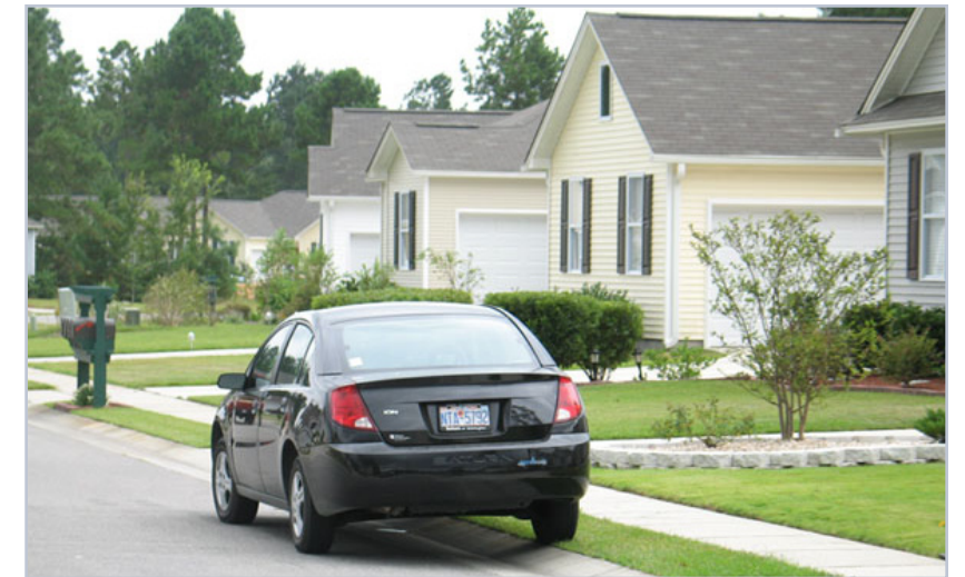
Overly narrow sidewalk (less than 4 feet)
