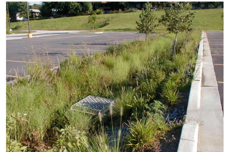
Rain garden with natural vegetation designed to capture stormwater run off from parking lot
