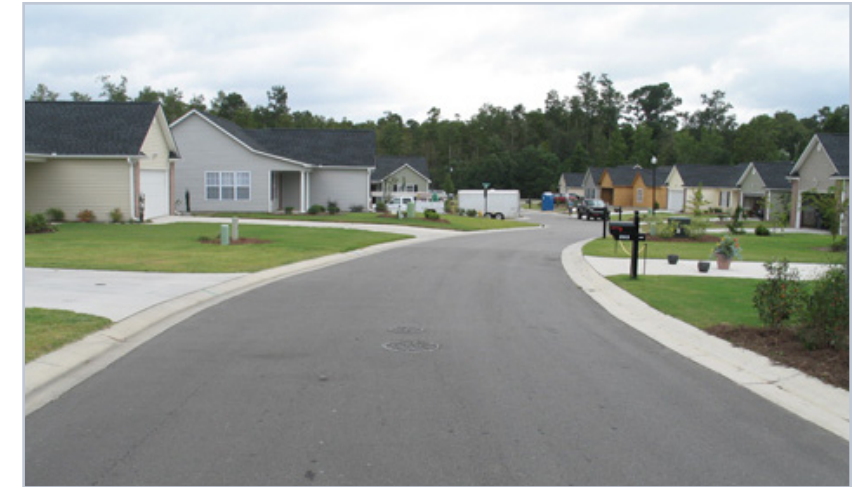
Overly wide subdivision street with no sidewalks or street trees
