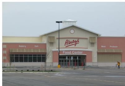
Limited landscaping in parking lot
