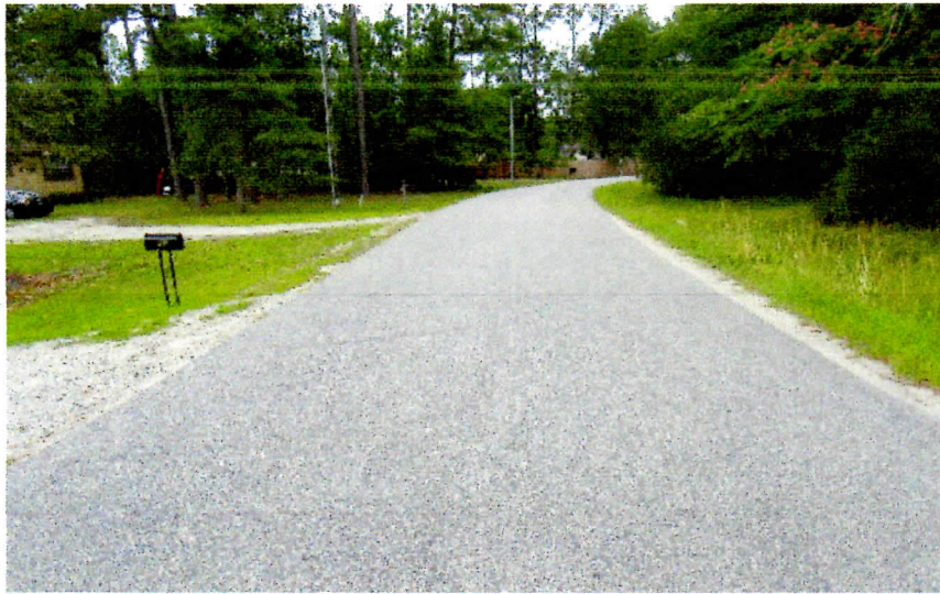
Figure 3 Rural Road Section
