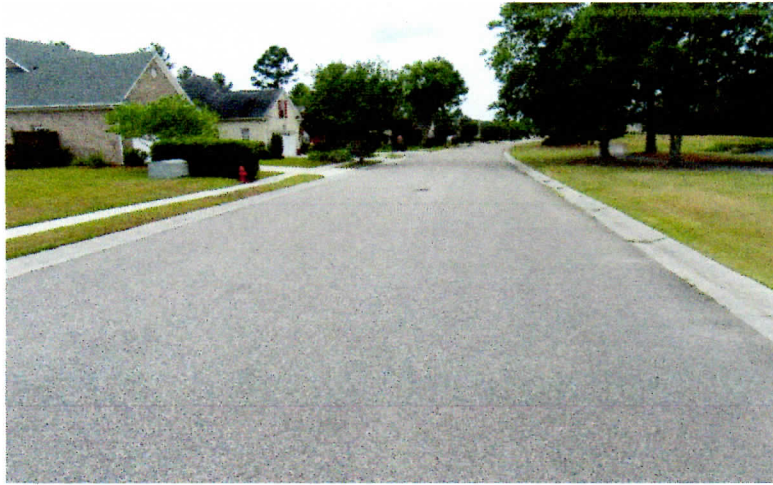
Figure 2 Rollover Curb and Gutter
