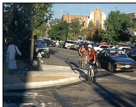
Horizontal —Bulb-out at an intersection
