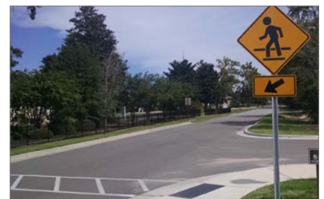
Pedestrian crossing with crosswalk, curb ramp, and signage (at Town Hall Dr).
