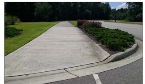
Multi-use path along Low Country Blvd.
