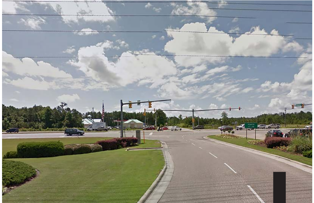
Right: Existing photo of Olde Waterford Way from the US 17 intersection facing east.
