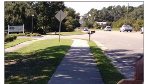
Typical 5'-wide sidewalk along Village Rd.
