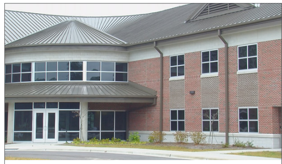
The new Leland Town Hall opened in 2015.
