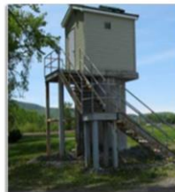
Wellhead Elevated above BFE (U.S. EPA)
