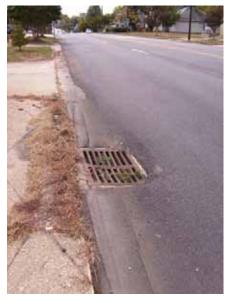
into a hole in the curb and have no slots on the road surface. Curb-face inlets offer an excellent solution, removing the grate entirely, however they can cause handling problems for bikes if the roadway slopes excessively toward the inlet.
