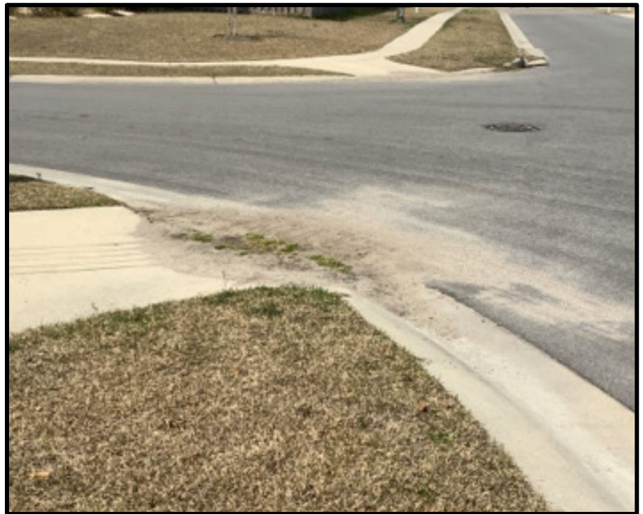
Island Pine Way @ Provincial Drive
